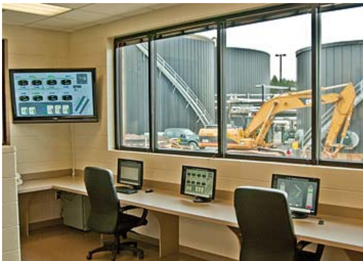
Terminal Office Computers are located at different places in the terminal in order to provide efficient control of all functions. For example: Positions of the three valves on the outlet side of each asphalt pump can be verified on a computer screen before the pump is operated. This view of the terminal office shows the user-friendly design and layout.
