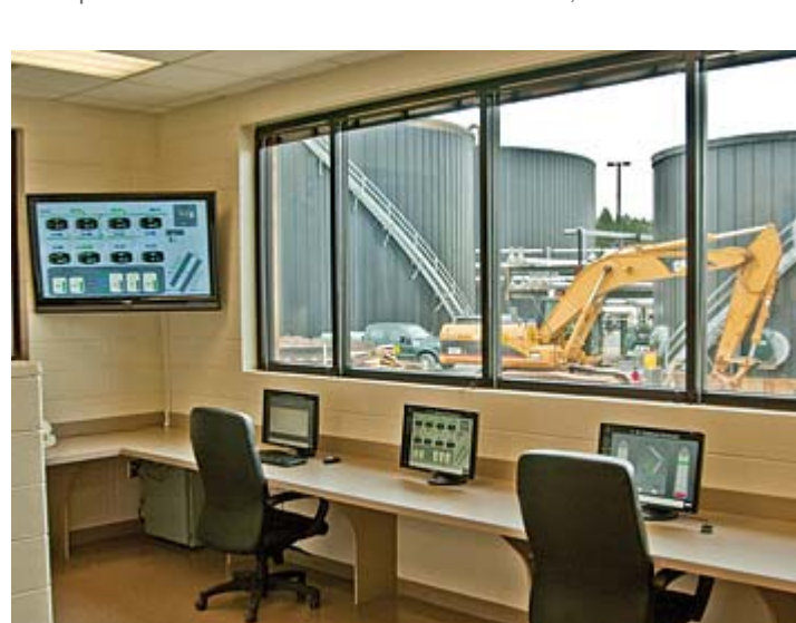
Terminal Office Computers are located at different places in the terminal in order to provide efficient control of all functions. For example: Positions of the three valves on the outlet side of each asphalt pump can be verified on a computer screen before the pump is operated. This view of the terminal office shows the user-friendly design and layout.
