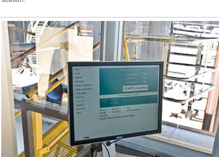
Computer at Load-Out Rack The load-out system incorporates a computer, computer-automated controls, two truck scales, and automated data recording. The automated controls provide remote operation of the asphalt pumps located at the tanks. The load-out controls for each load-out boom incorporates lockouts to prevent operation of the pumps unless the boom is properly positioned and valves are properly set. The components of the truck scales and the load-out system were provided by Astec.
