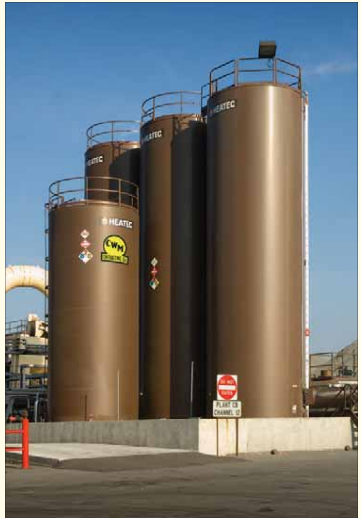
Here is another view of the company's Kennesaw, Georgia facility. This one focuses on the Heatec vertical storage tanks for liquid asphalt cement.
